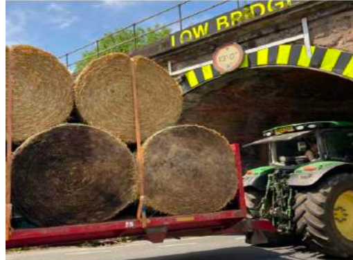
Photo 6 Pinch Point under Railway Bridge
