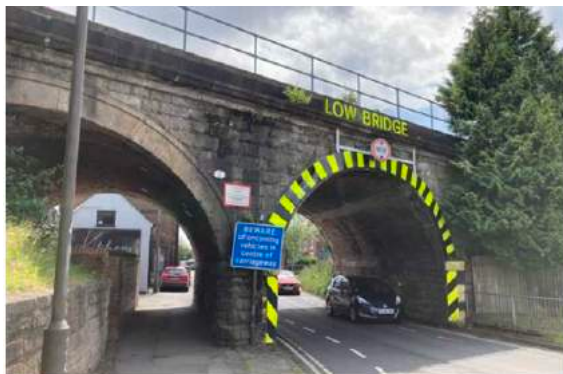
Photo 5 One of two routes under the railway
