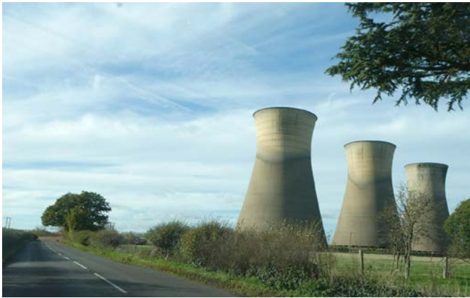
Figure 26: Approach from the East towards Power Station
