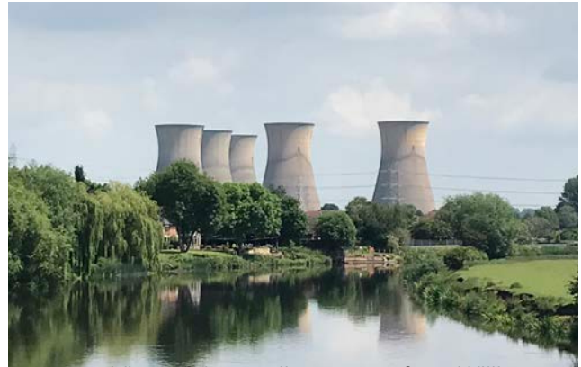
Figure 88: View of the cooling towers from Willington Bridge
