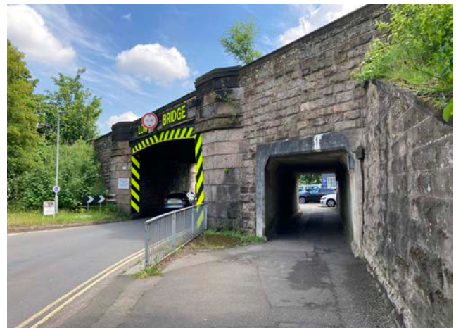
Figure 65: Vehicle and pedestrian gateway through pinch point
