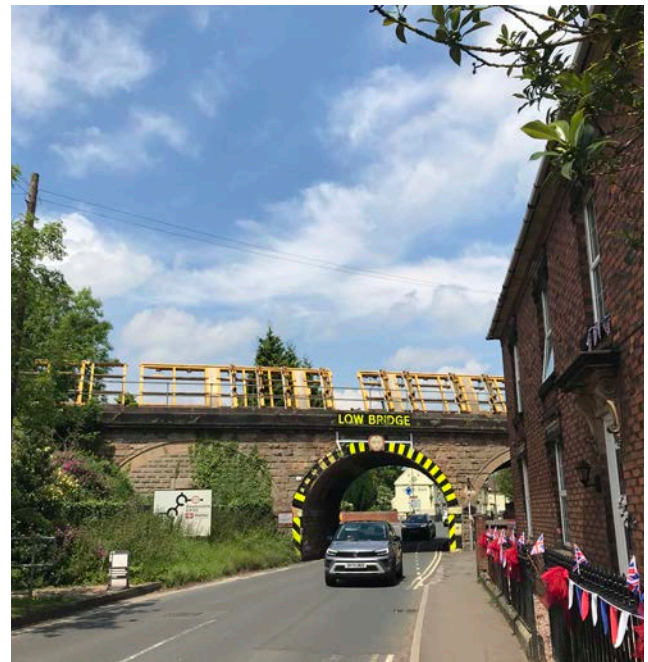
Figure 49: Repton Road (looking north towards railway)
