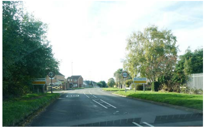
Figure 27: View approaching from the east from the Village entrance
