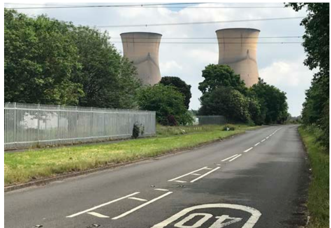
Figure 89: View of the cooling towers from Twyford Road
