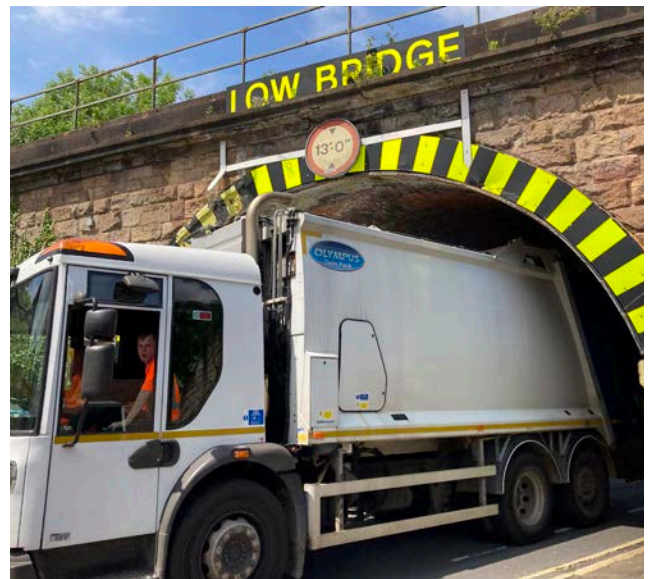
Figure 66: Pinch point potentially causes congestion due to slow moving traffic
