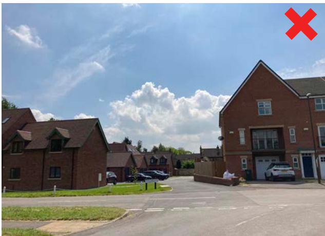
Figure 105: Front of property parking detracts from prevailing character in this location.
