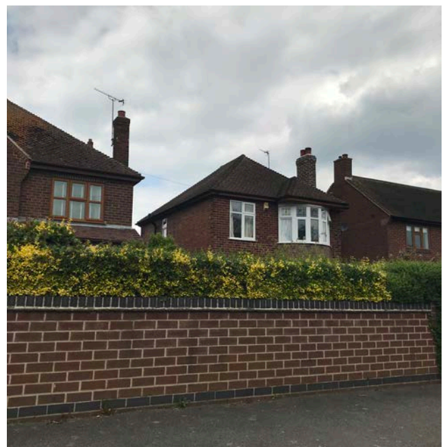
Figure 76: a mix of roof and boundary types
