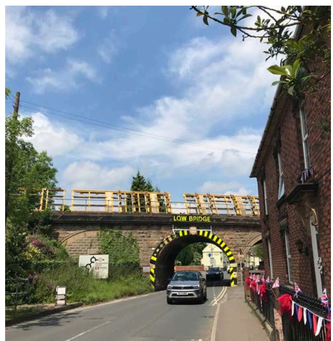
Figure 38: Tunnel under railway line
