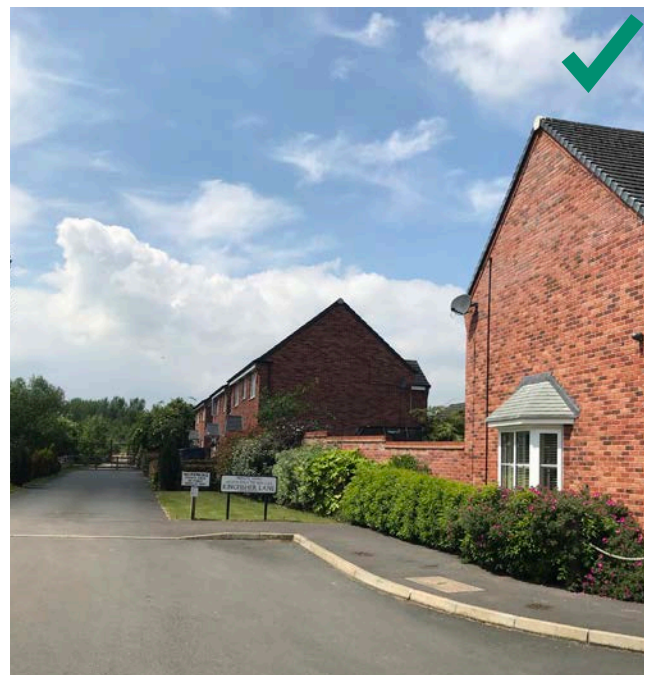
Figure 126: Corner turning properties or dwellings that front both sides aid in site legibility
