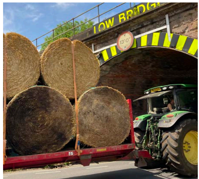
Figure 62: Pinch points for both pedestrians and vehicles
