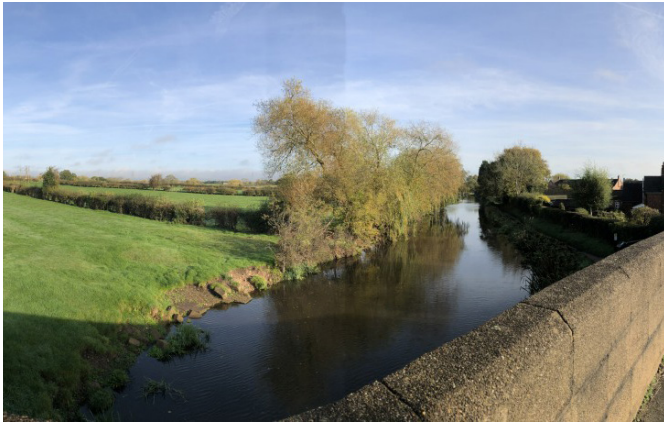
Figure 24: View N/NE from canal bridge
